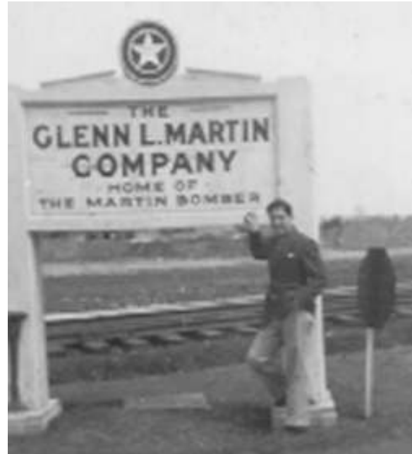
Fig 19. Entrance to Glen L. Martin Plant
